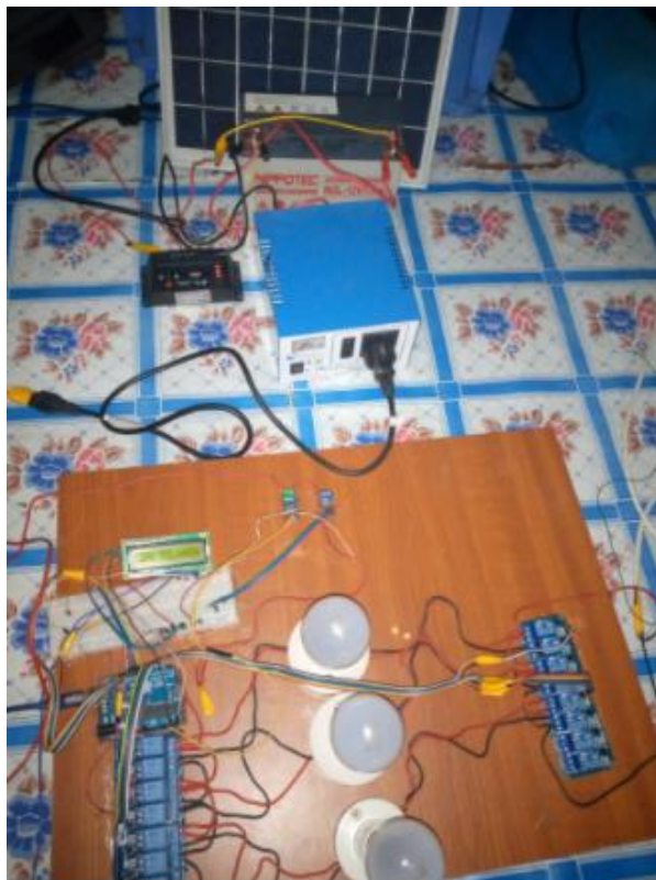
Figure 8. Snapshot of assembled hardware components
