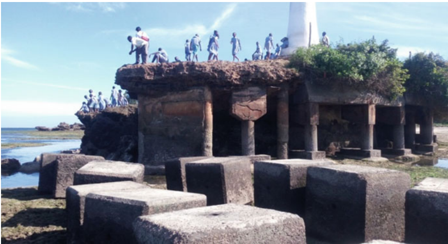
Fig. 3 Vasco da Gama Pillar in Kilifi
