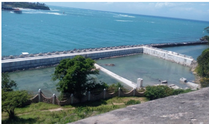
Fig. 4 Construction of sea wall at Fort Jesus (Authors 2019)
