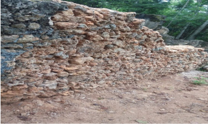
Fig. 5 Repaired wall at Gede Ruins (Authors 2019)
