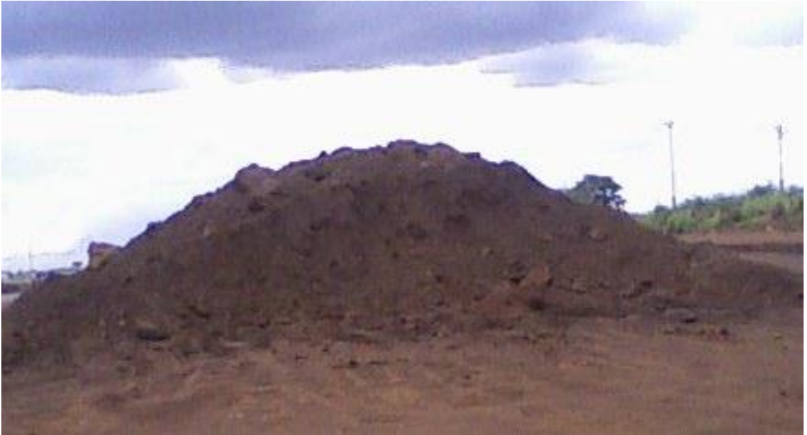
Plate 2. 1 Laterite being used in construction of the Thika Super Highway
